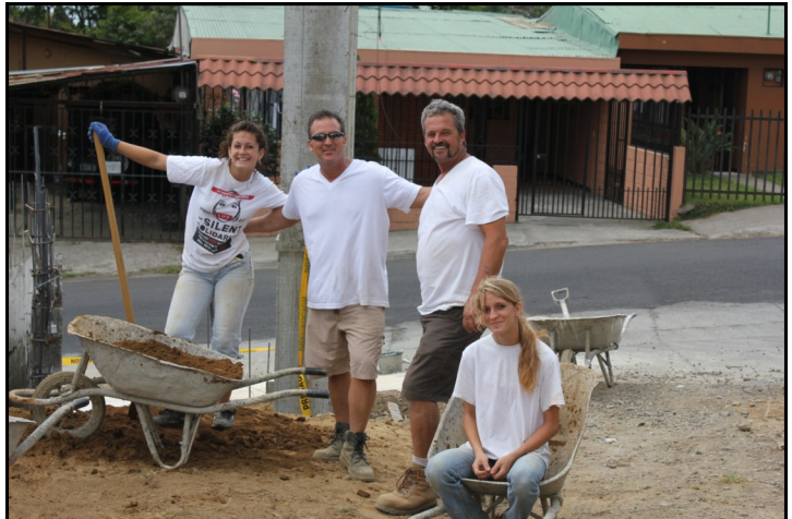
Work begins on the front gate at the Children's Home
