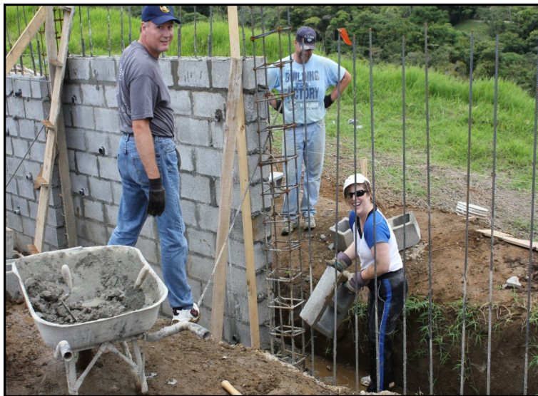
Work continues on the retaining wall for house #2
